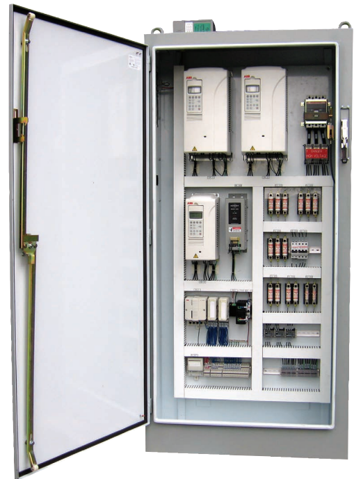
Control Cabinet for Winches
